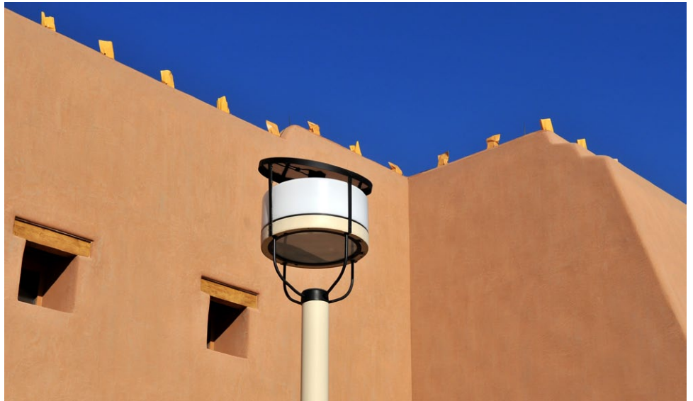
A pole light with Noribachi's LED and solar custom lighting retrofit at Sandia Resort & Casino
